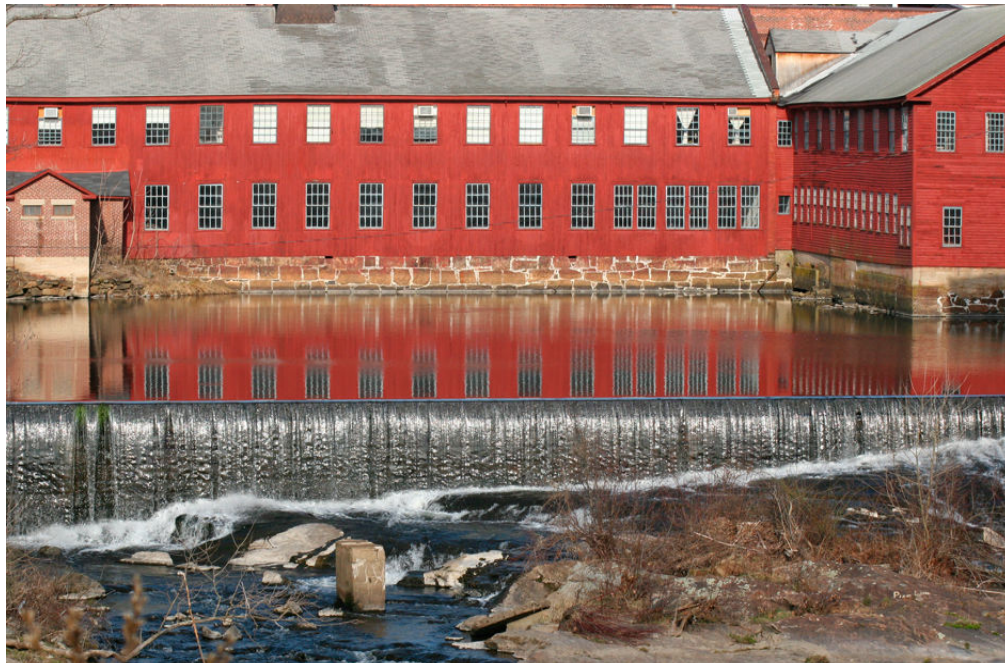
HATCHET FACTORY & DAM – FRANK JAMES
